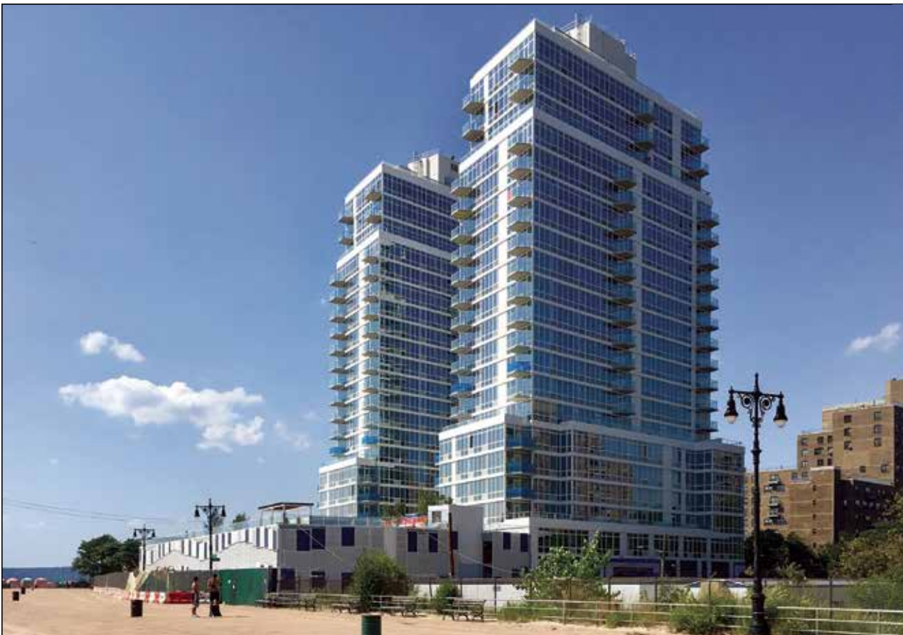
Billionaire John Catsimatidis is building the upscale Ocean Dreams apartment complex on the Coney Island Boardwalk. Would he consider paying to fix up the damaged walkway? INBrooklyn photos by Lore Croghan
